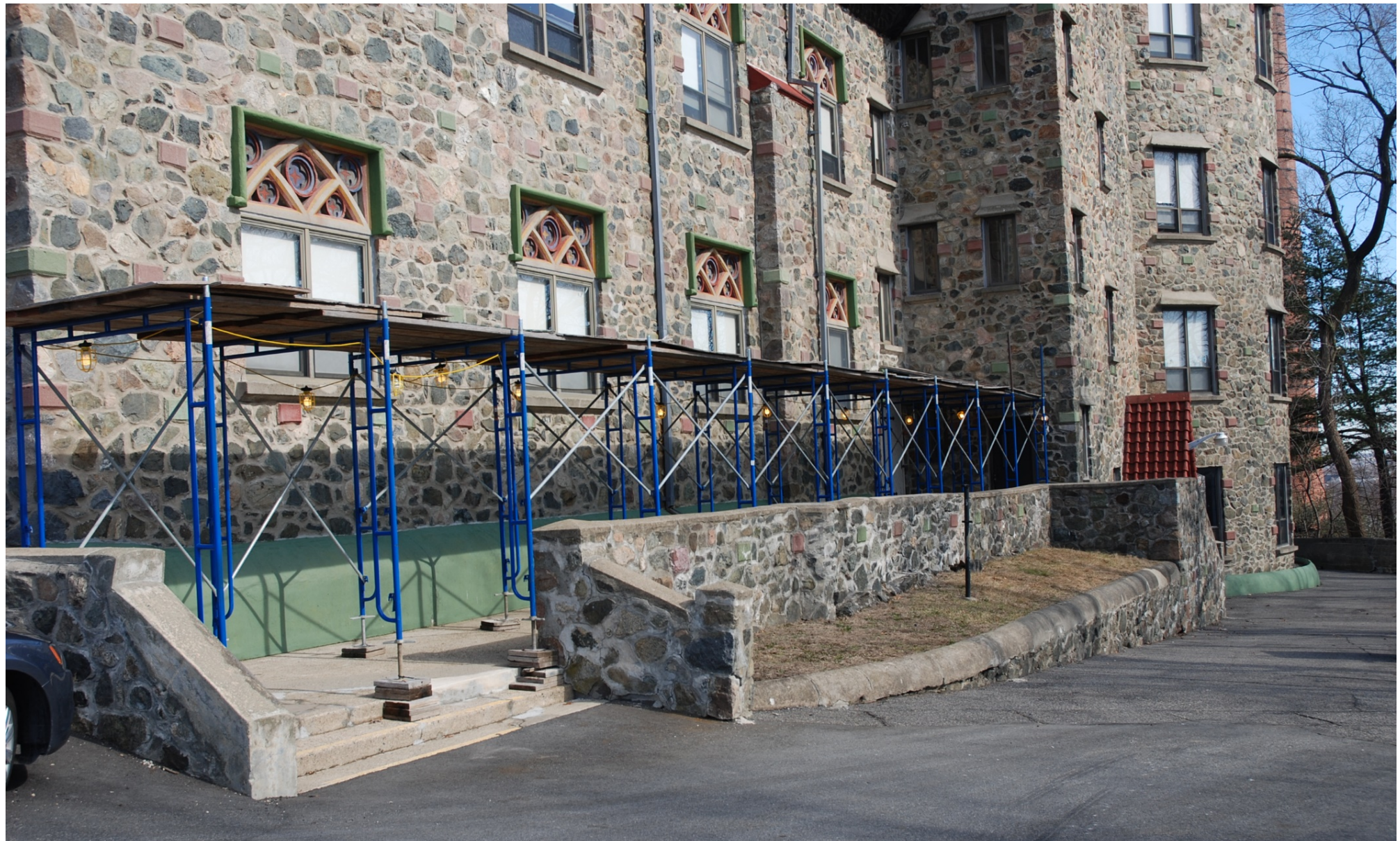
View of protective scaffolding at Tower A walkway
