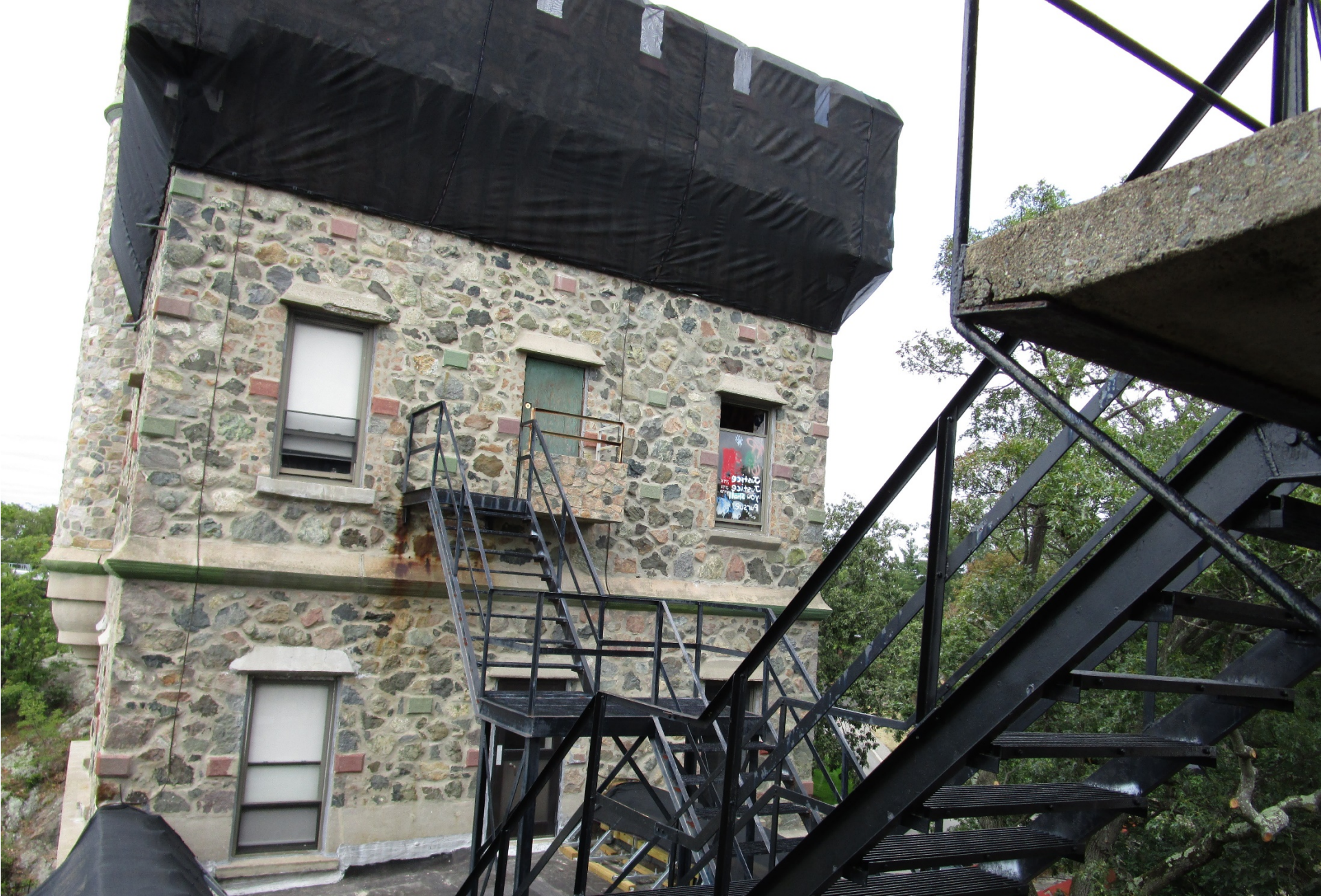
View of rooftop fire escape at Tower A
