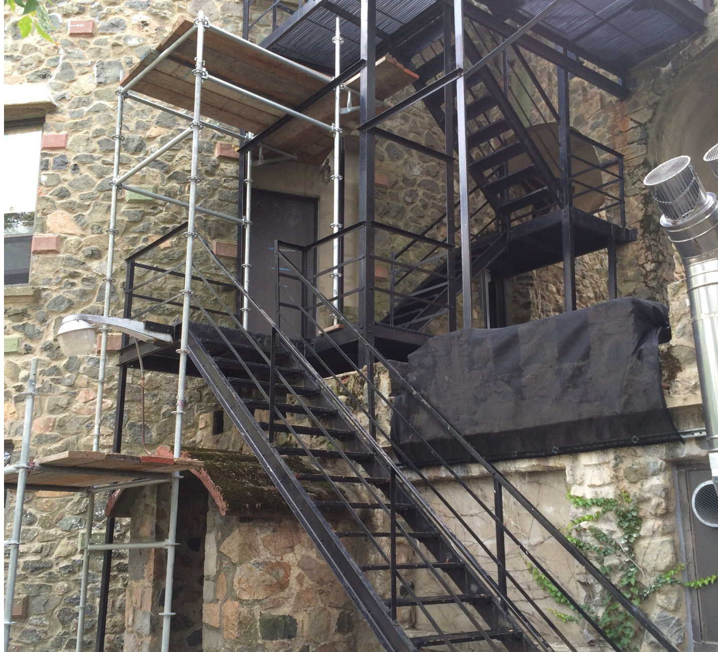
View of fire escape and protective scaffolding at Tower B
