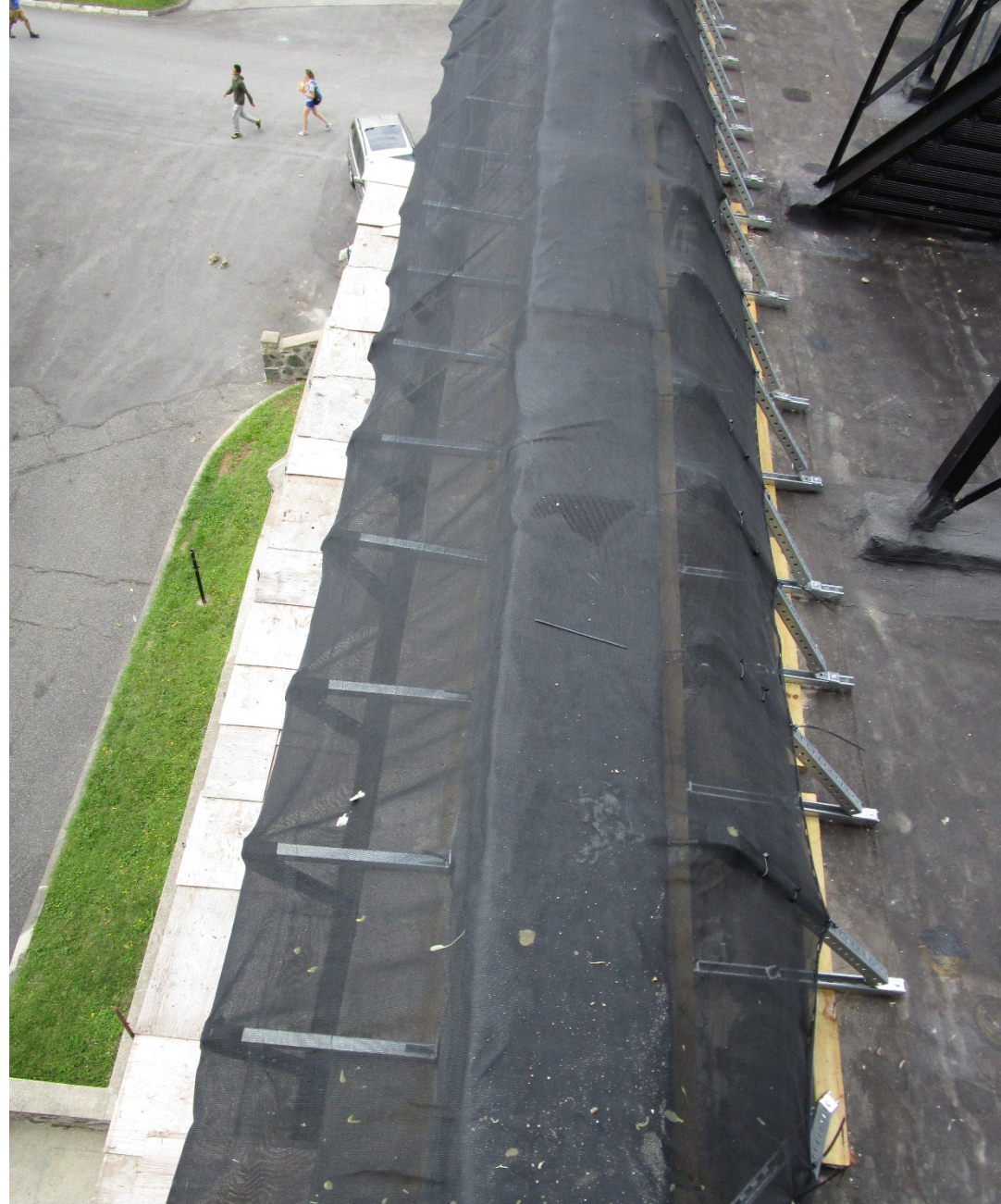
View of added bracing and protective netting at Tower A roof
