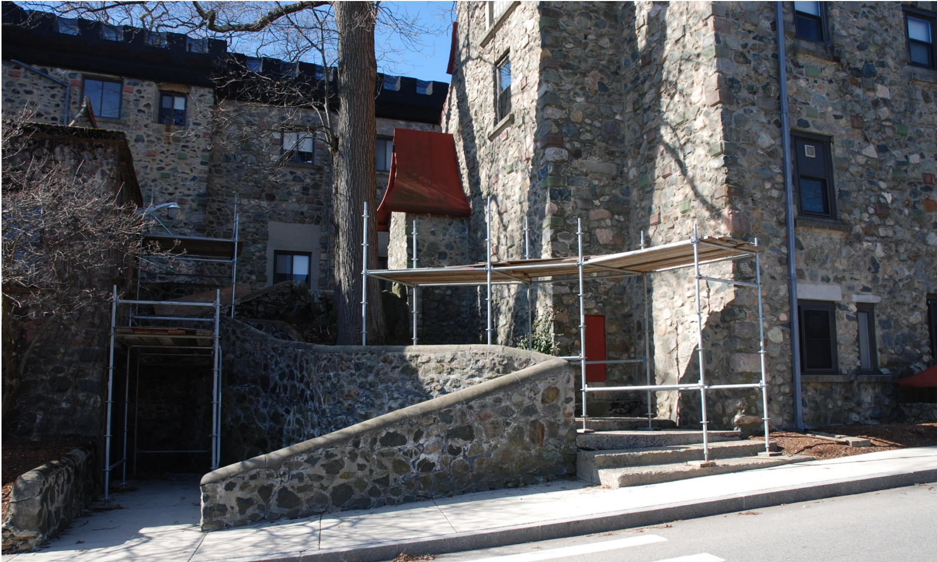
View of protective scaffolding at Schwartz Hall walkways
