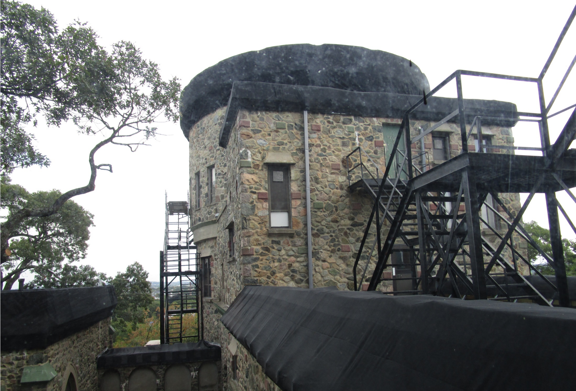
View of rooftop fire escapes at Tower B
