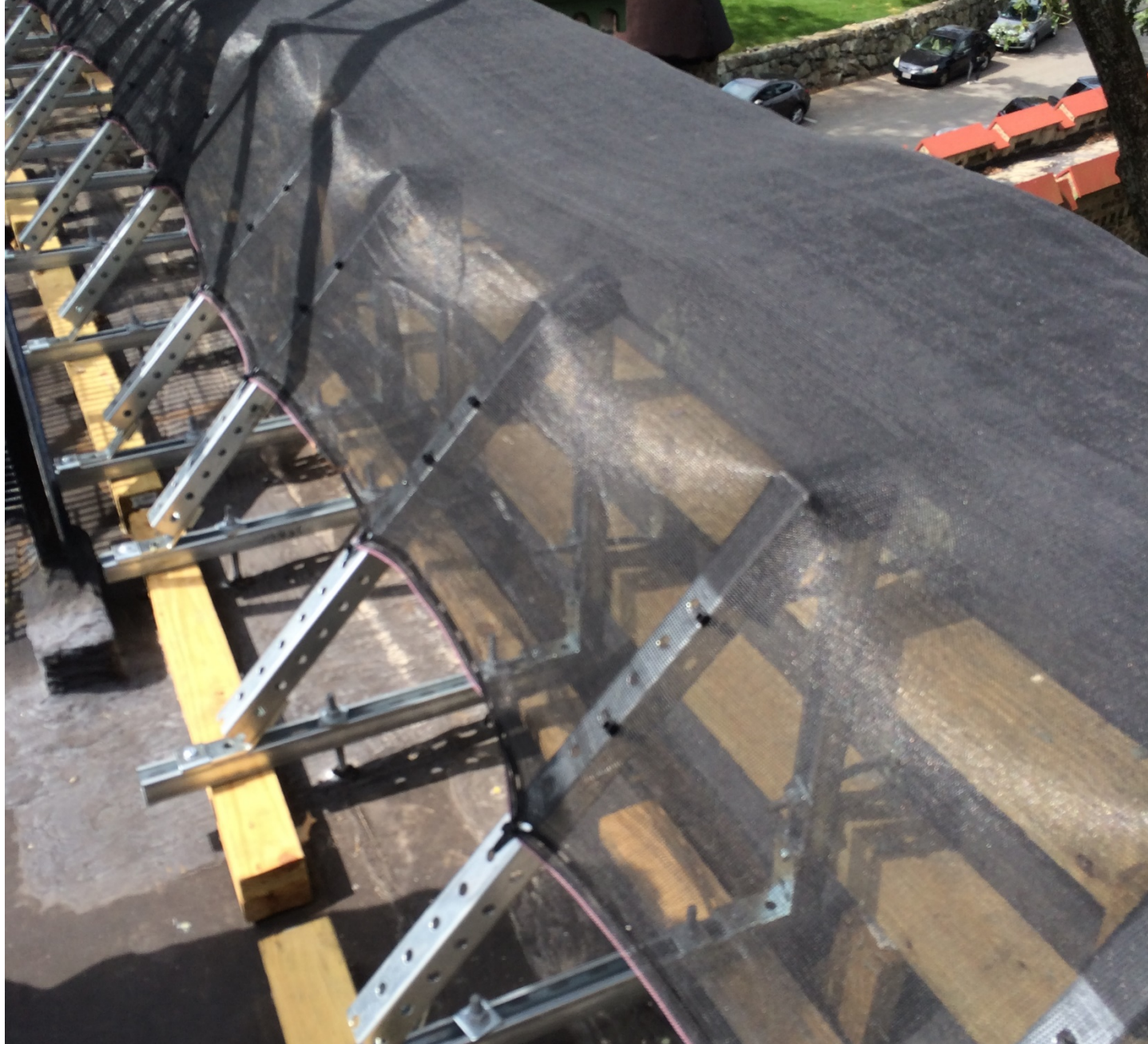
View of added bracing and protective netting at Tower A roof
