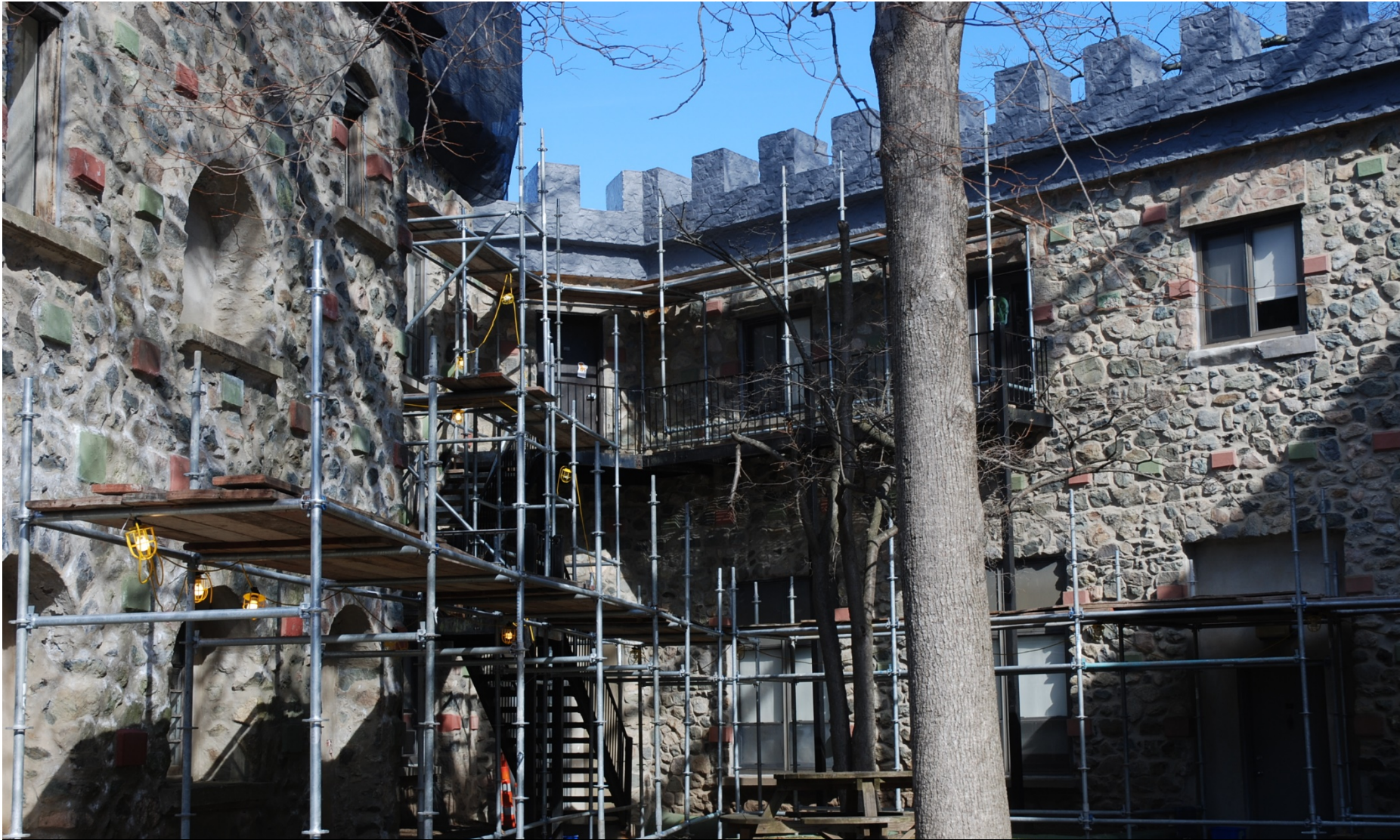
View of protective scaffolding in courtyard
