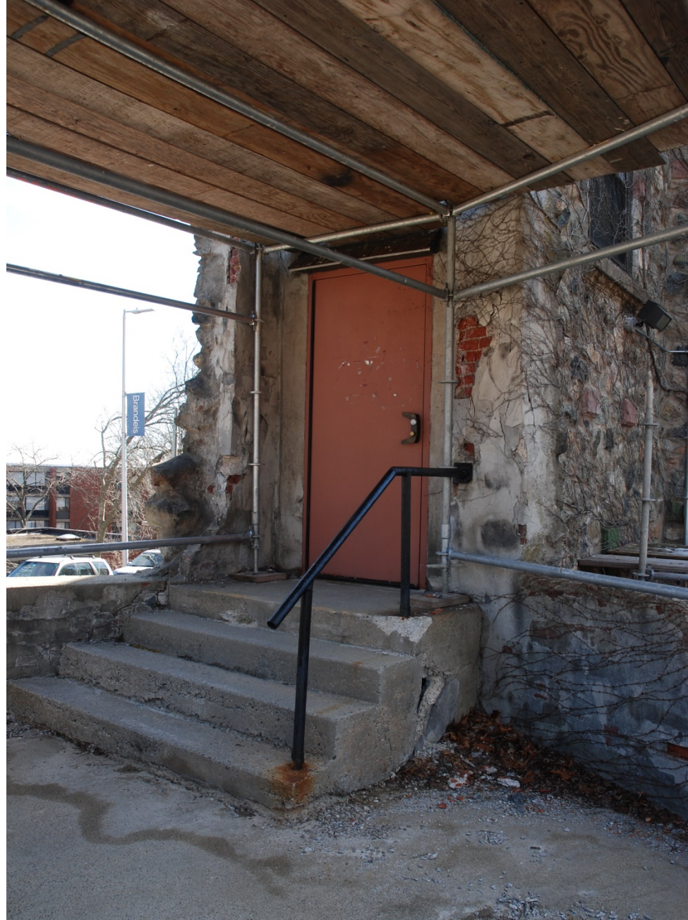
View of protective scaffolding at Schwartz Hall entry
