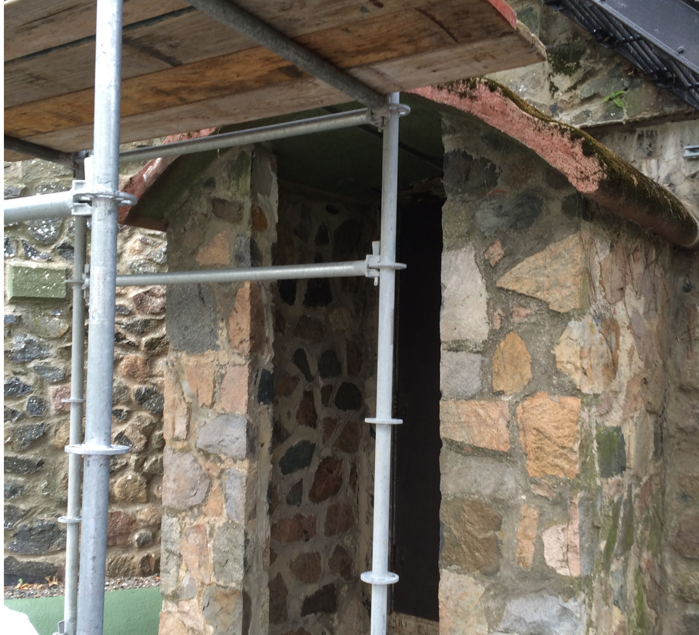
View of protective scaffolding at Tower C entry
