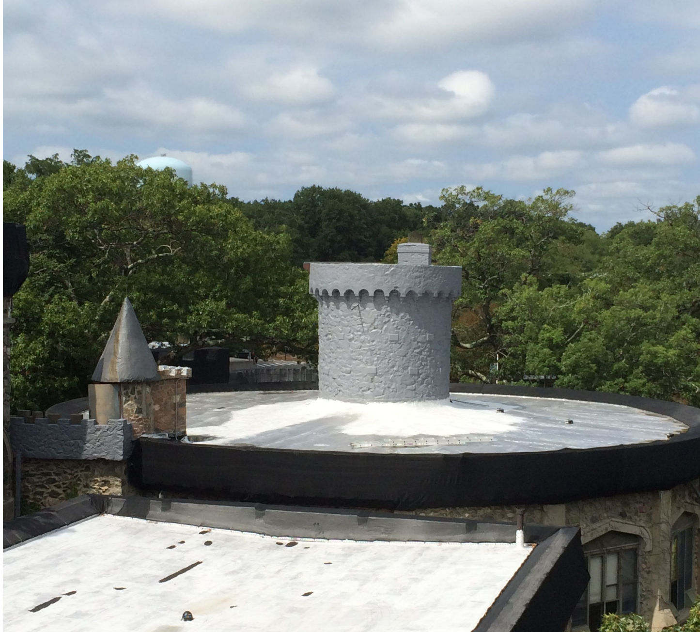
View of the roofs at Tower C and Tower D
