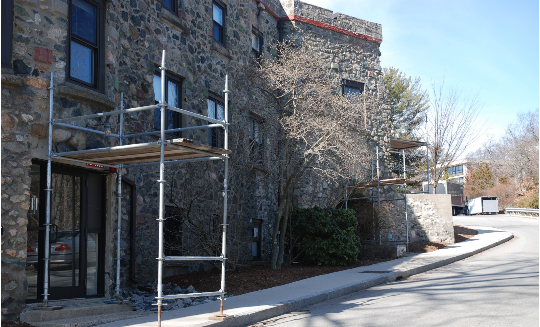
View of protective scaffolding at Schwartz Hall entries
