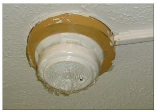
Smoke Alarm...also often known as smoke detectors, these devices are one of the best early-warning devices of a fire. They are designed to sense low levels of smoke and sound an alarm.
