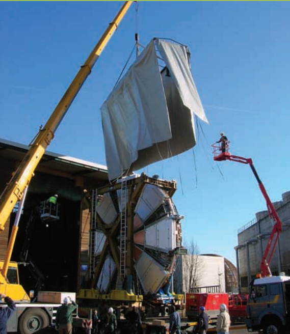
Small wheel developed and built by Brandeis and other area universities is unveiled for the ATLAS experiment in the Large Hadron Collider.
