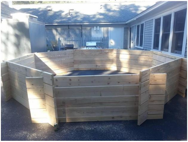
The Gaga Pit ended up fulfilling all of the design constraints: it is mobile because it can be taken apart and put back together. It is sturdy enough to handle kids leaning and sitting on it, and can be easily assembled and disassembled by others with very little instruction.
