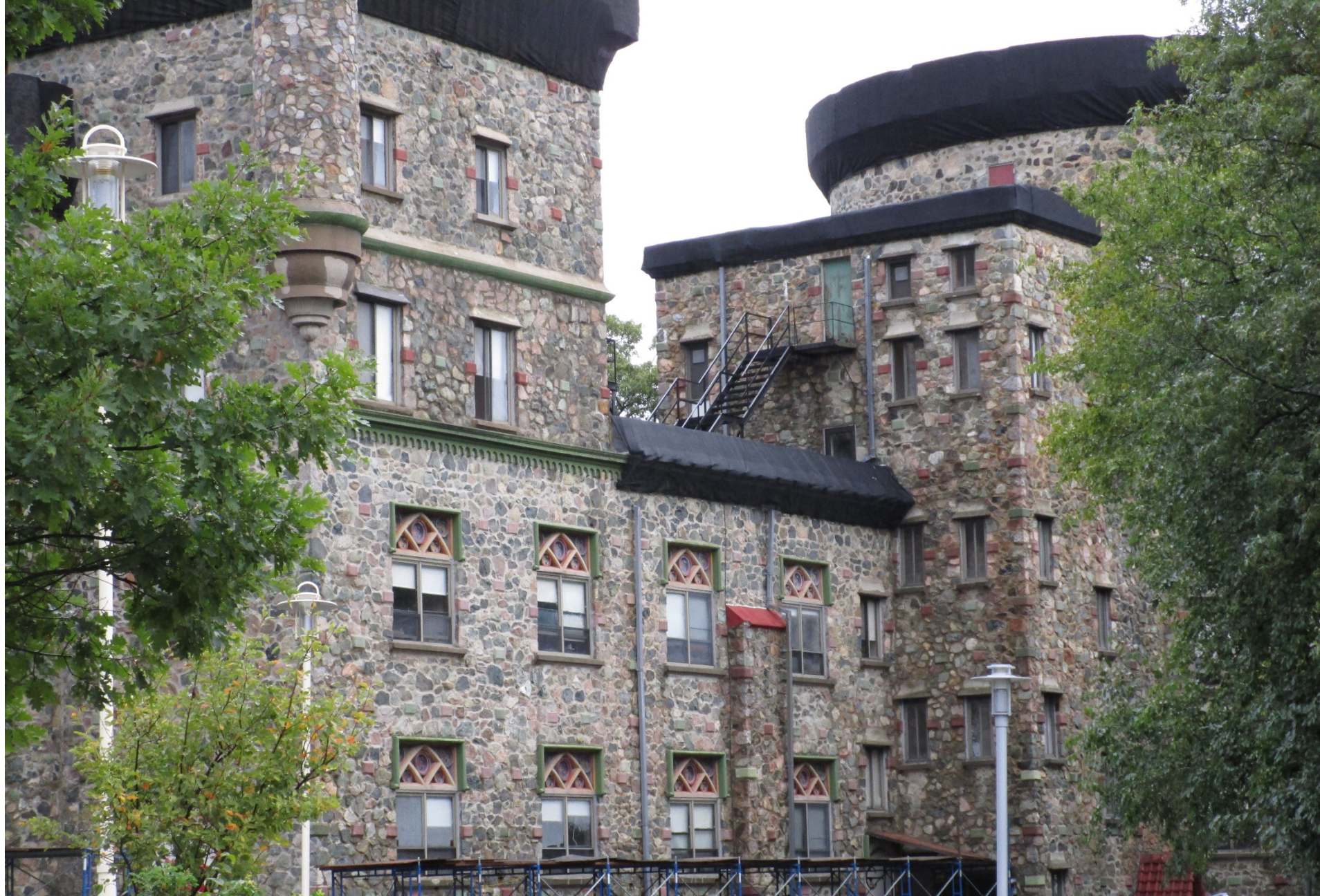
View of protective netting at parapet, scaffolding at walkways & rooftop fire escape at Tower A and Tower B
