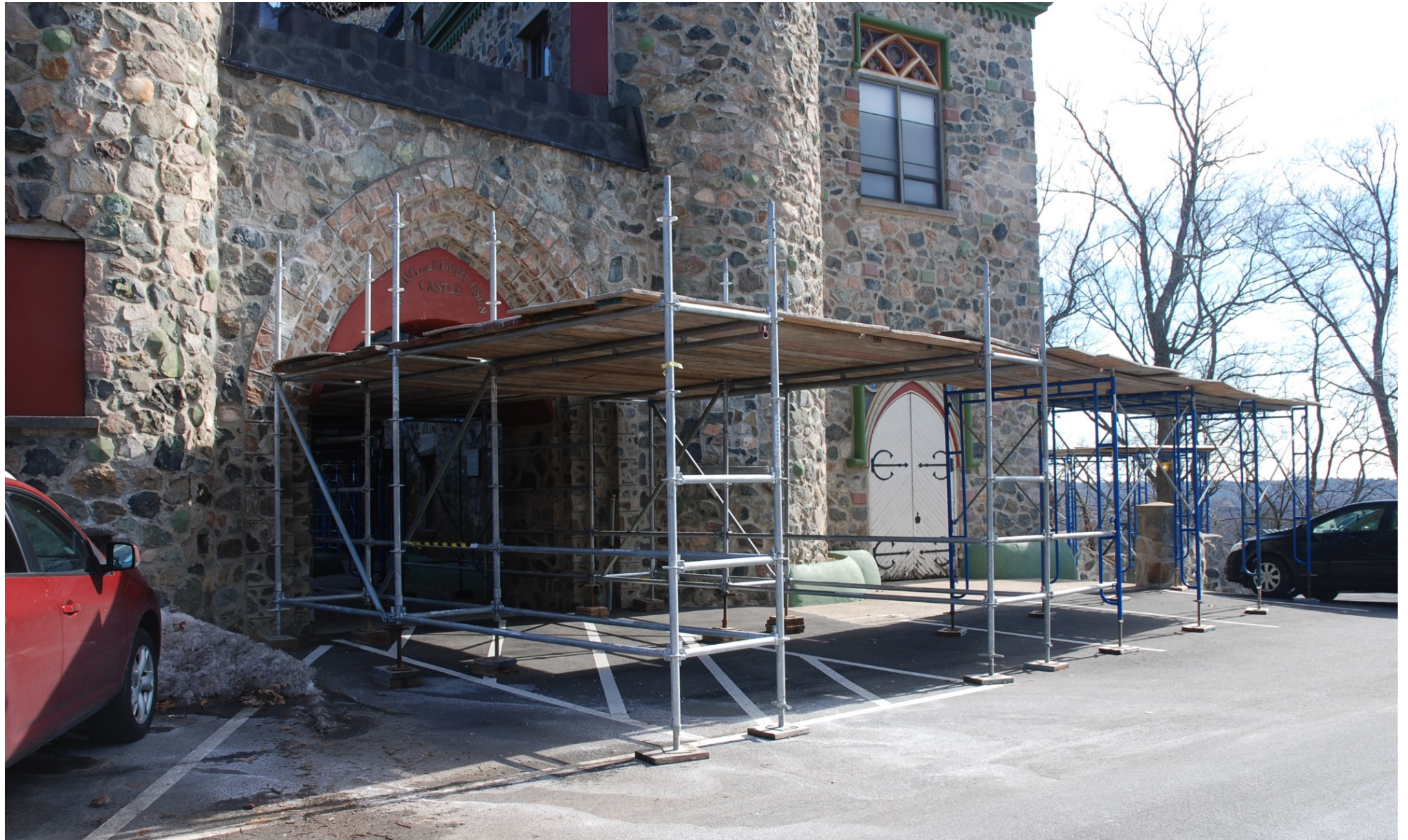
View of scaffolding protection at courtyard entry
