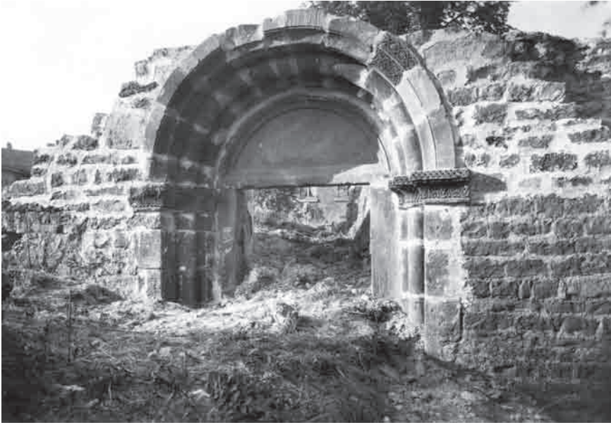
FIGURE 34. Photo of the erected portal (1949). Stadtarchiv Worms, Germany
